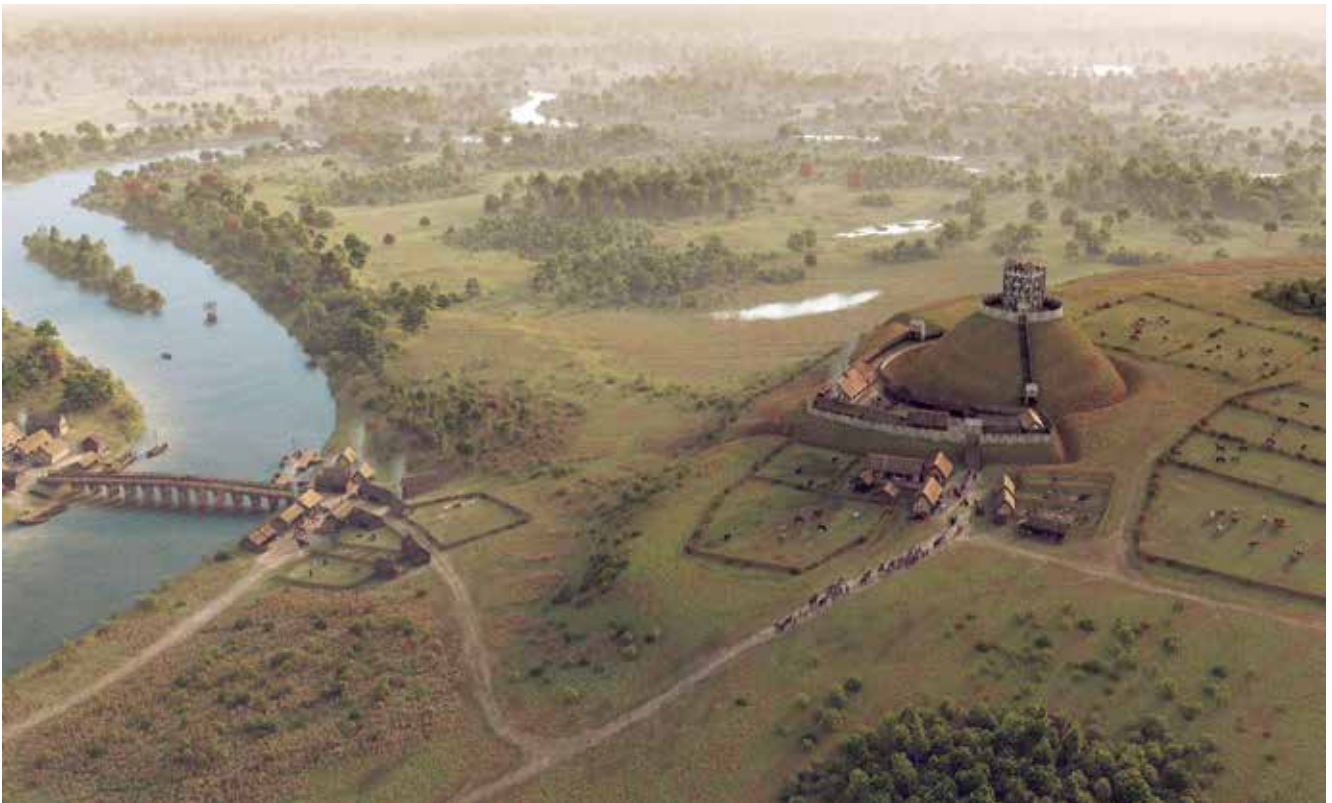
Fig. 1: A conjectural reconstruction of Windsor Castle c. 1100. The castle was built as a 'motte and bailey', with earthwork defences and timber buildings. Reconstruction by Bob Marshall.
