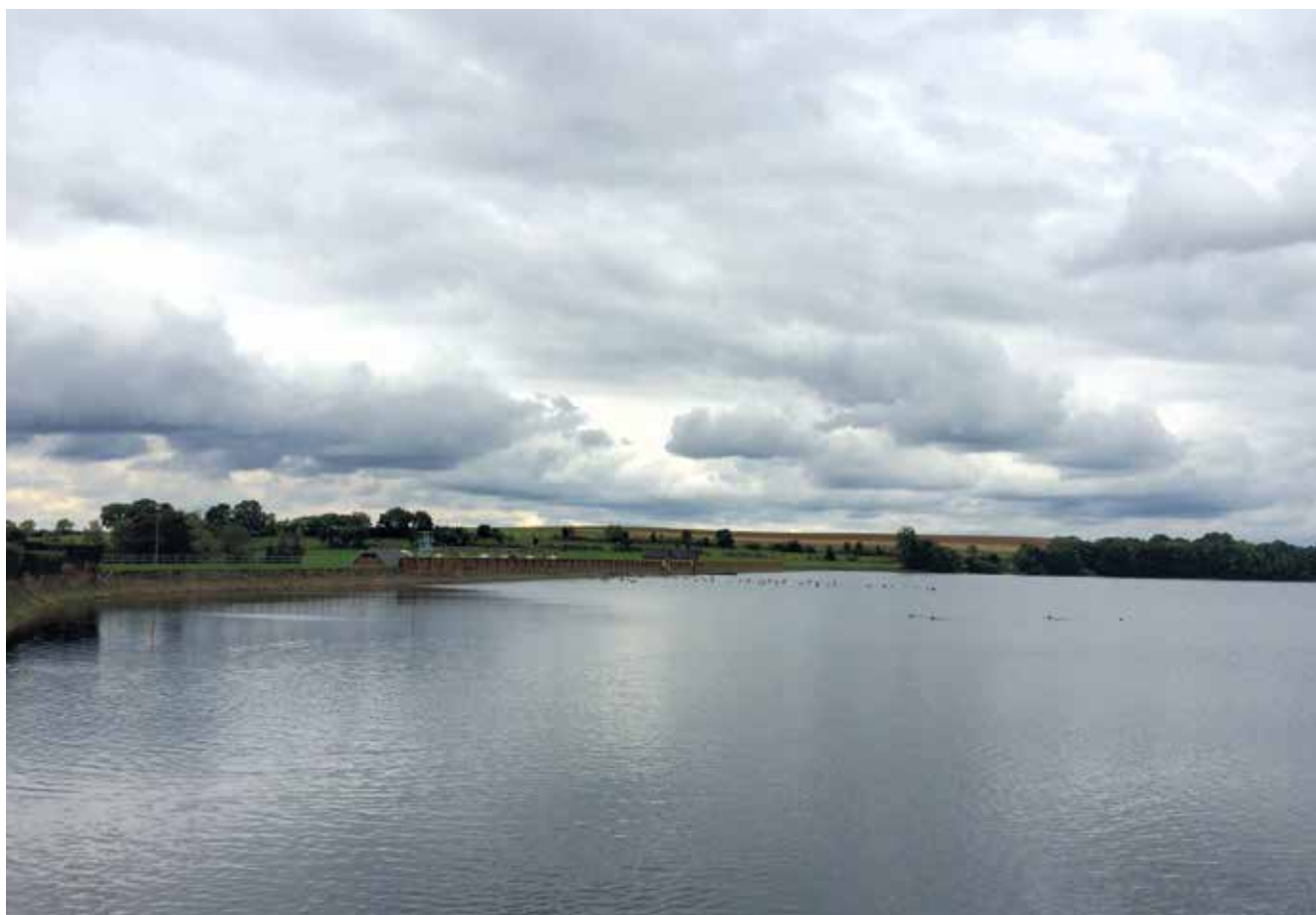
Fig. 7: Water management system, Großhartmannsdorfer pond, Freiberg mining landscape (photo: Friederike Hansell, IWTG)
